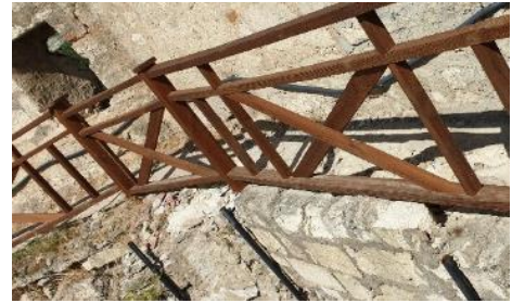
A child can fall through the mesh of the railing
