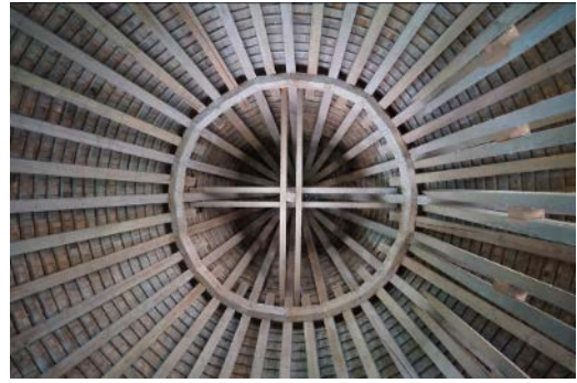
Soroca fortress roofs: wooden structures consisting of a warp of beams covered with wooden tiles
