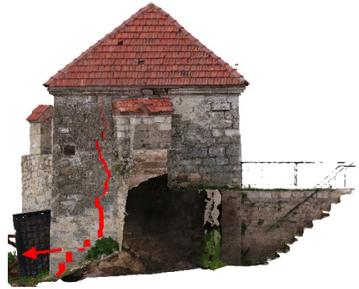
Rotation at the foot of the wall due to ground subsidence
