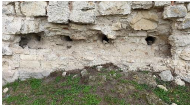
Collapse and local loss of the stone face at the voids left by the lost wooden net
