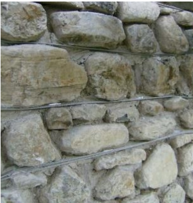
The steel strands inserted inside the mortar joints and the joints after the proposed intervention.
