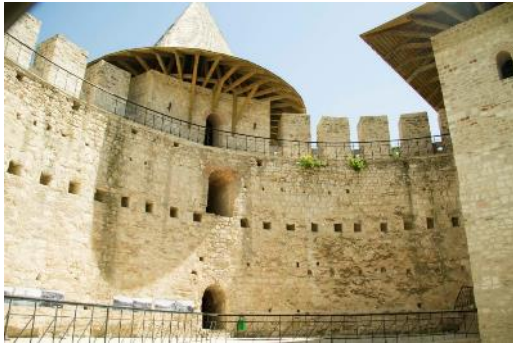
Soroca fortress roofs: wooden structures consisting of a warp of beams covered with wooden tiles
