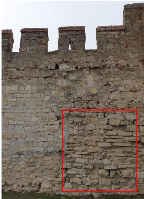
Loss of joints, degradation of stone facing, loss of stones
